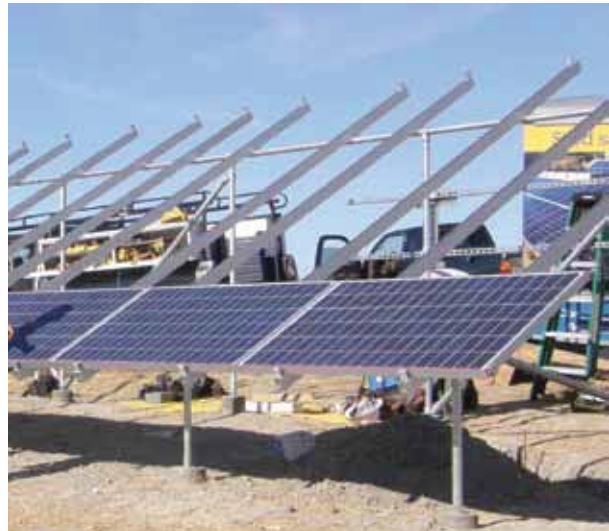
First row of modules installed
