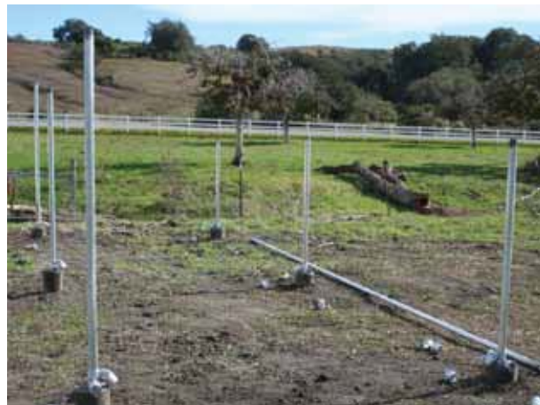
Install vertical pipes in concrete footings
