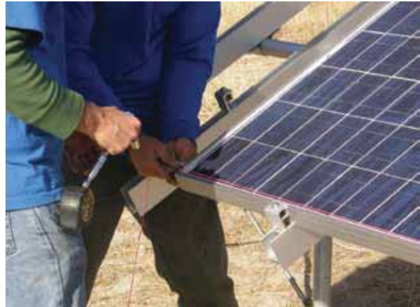
Aligning first row of modules
