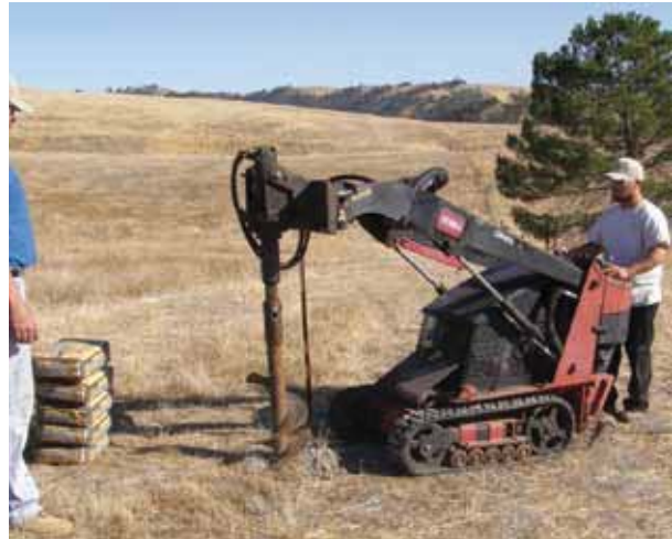
Digging holes with power auger
