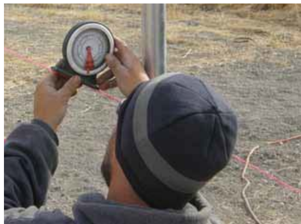
Check pipe frame levels
