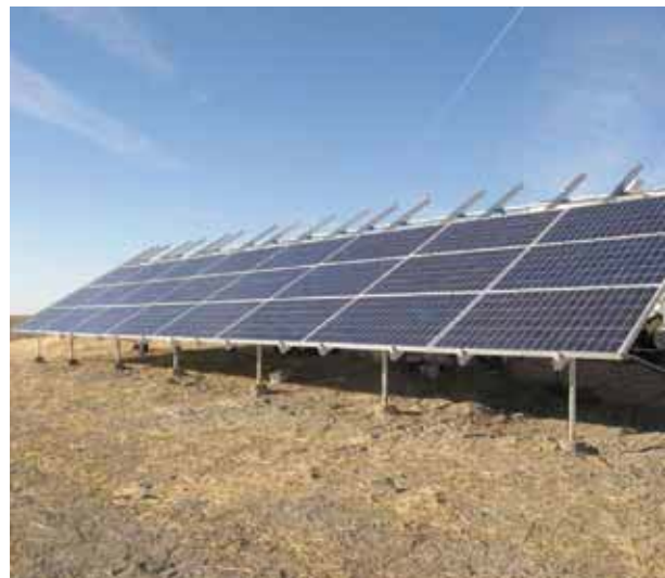
Three rows of modules installed
