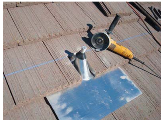
Install flashing using appropriate methods for roof type. Slide rain collar over flashing.
