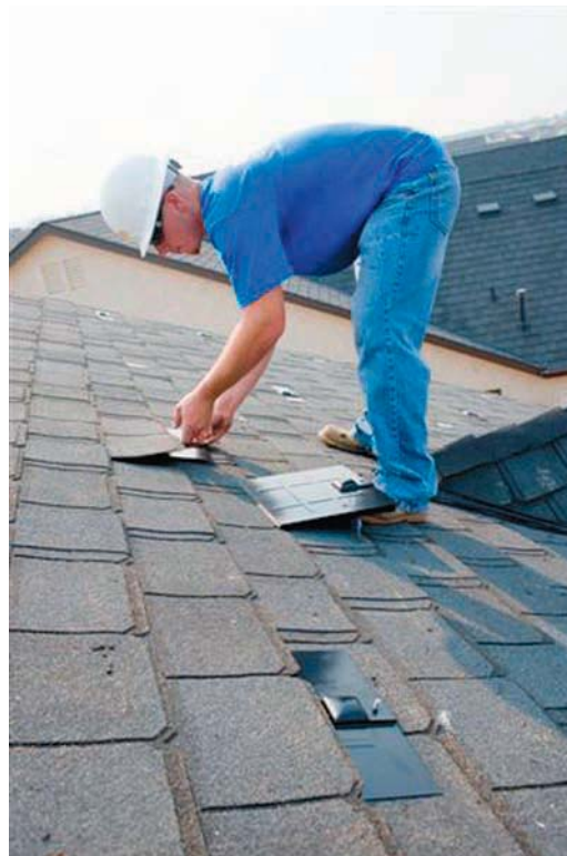
Install flashing
