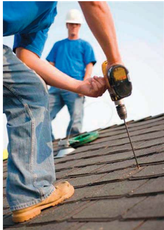
Drill pilot holes
