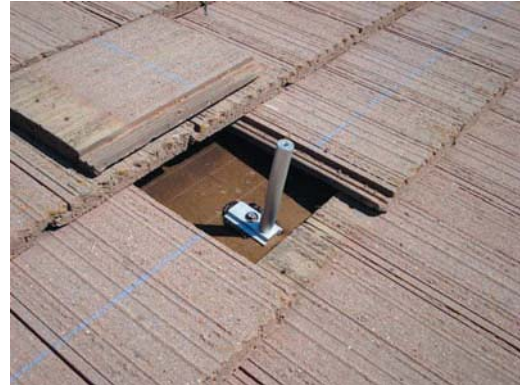
Screw standoff onto base
