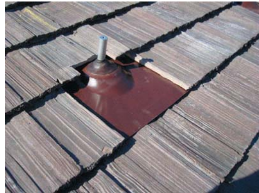
Standoff installation using Oatey flashing
