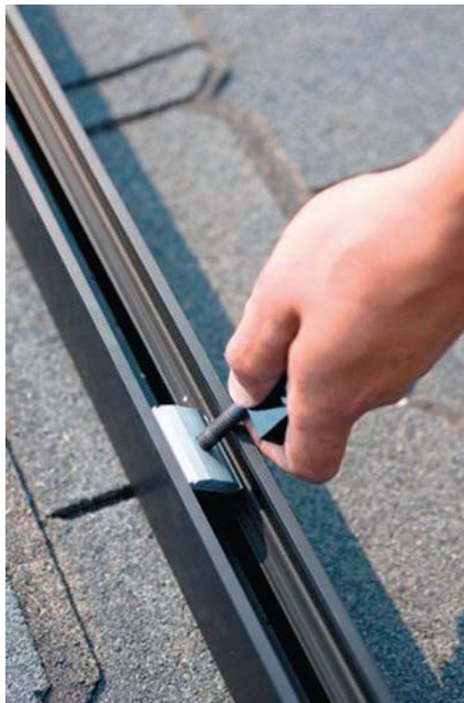
Snap module clamp assemblies into rail
