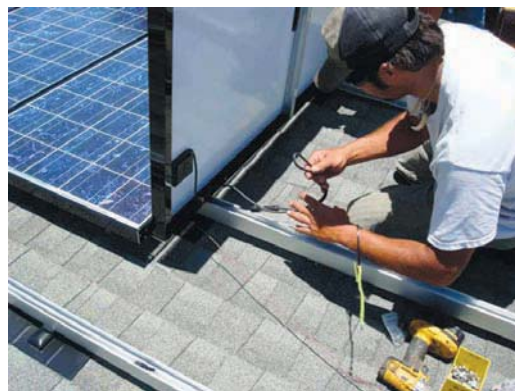
Connect wiring
