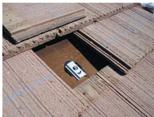
Typical standoff base installation
