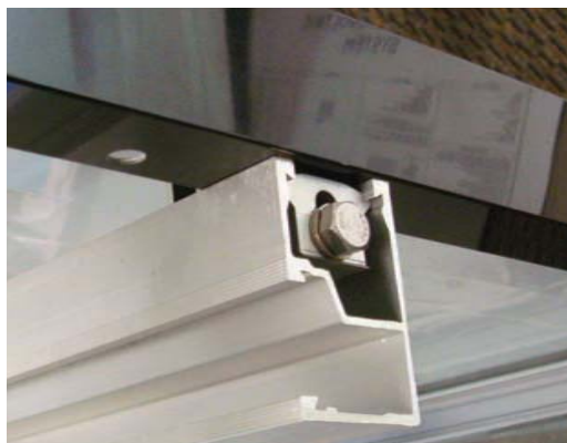
Installed Universal End Clamp
