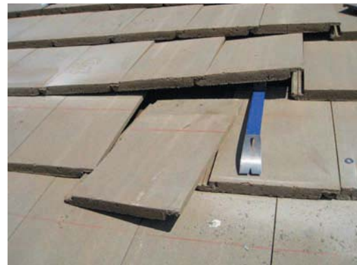
Remove roofing material to expose roof underlayment
