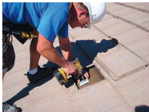
Secure standoff base to rafter
