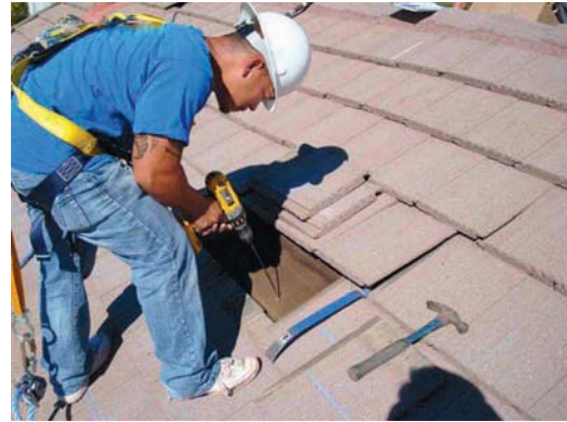
Drill pilot holes
