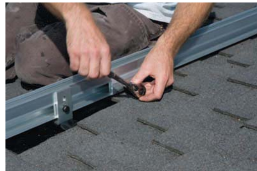
Tighten bolts on splice
