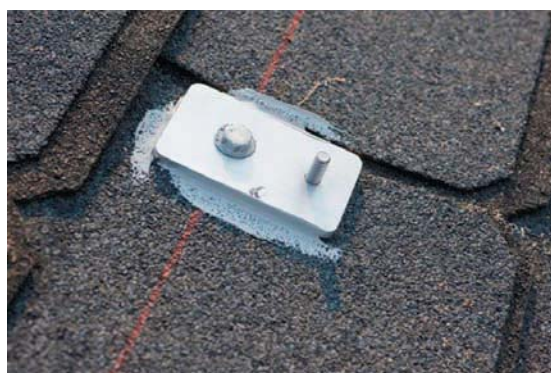
Apply sealant and secure base to rafter
