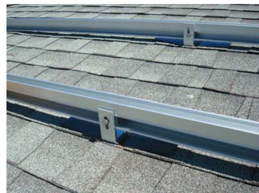
Standard rail mounting configuration
