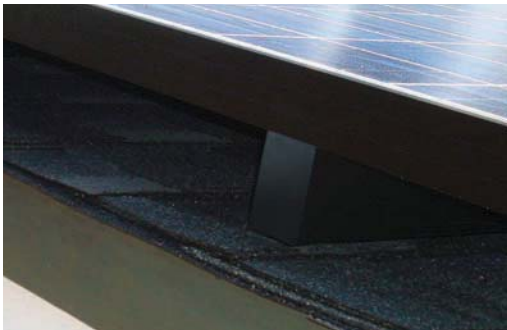
Rubber end cap installed
