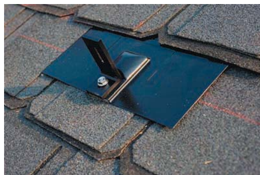
Installed L-foot assembly
