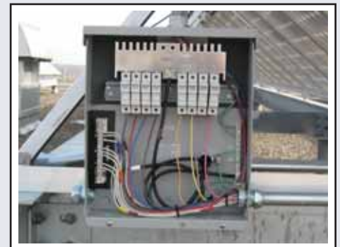
MNPV12 installation Photo by Darryl Thayer
