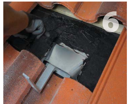
After first layer of cement is dry, apply second layer over reinforcing fabric to finish waterproofing of sub-flashing.
