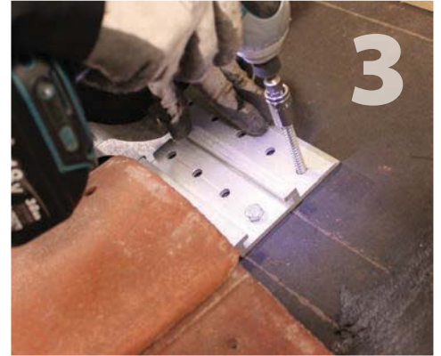
Connect hook to base plate and drive lag screws into rafter through the two holes to a solid, snug fit. DO NOT over tighten lag screws, this may compromise their holding strength.
