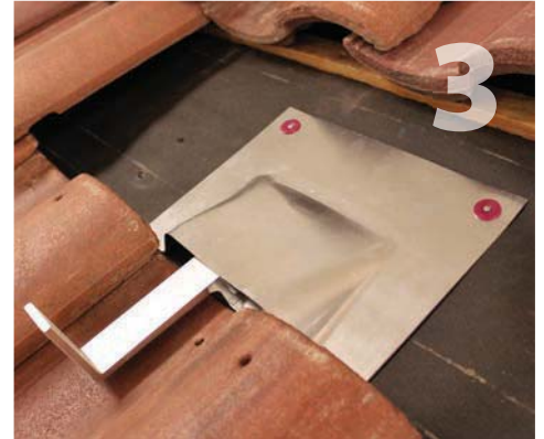
Install the sub-flashing over the base and hook. Fasten the sub-flashing into place with two roofing nails, one in each top corner. Clean away dust and debris.
