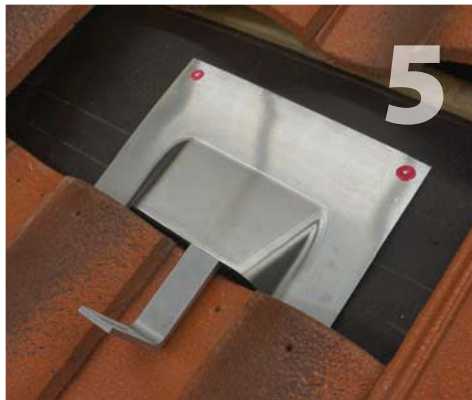
Carefully clean the underlayment then apply bead of sealant compatible with roofing materials in the shape of an upside down U on the backside of the sub-flashing, see example on page 2, and install flashing over mount. Fasten sub-flashing to deck with one roofing nail in each top corner. Do not nail bottom corners.
