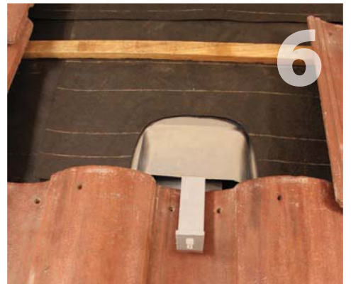
Flashing must be sealed to deck using three-course method with mastic and mesh, see page 2, or underlayment bibbing. When bibbing, the upper edge of the bib should extend 3" under the course of underlayment above the flashing and the bib should be wide enough to overlap the sides of the flashing by 3".
