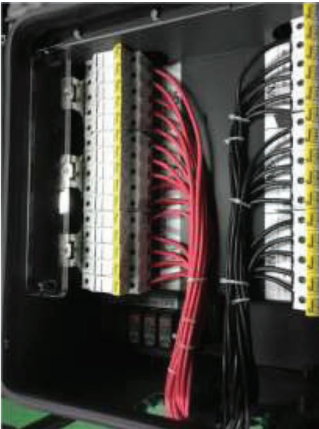
Figure 2.21- DC Input Cable Connection
