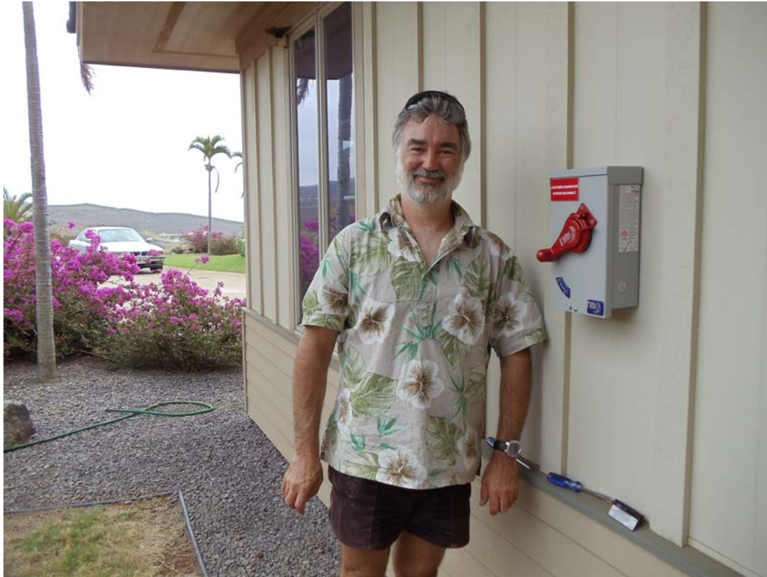
Figure 7 Our happy installer, Tom Carpenter.
