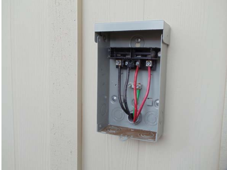
Figure 3 Square D pull switch wiring. The shorting bar has been removed. Leg1 in and out on the left (black) and leg2 in and out on the right (red). The shorting bar (pull bar) has two pieces of brass that connect the ins and outs together when installed. This meets code, but is not very handy. You must first unscrew the cover, then pull real hard to get the switch disconnected. Not what you would want to go through in an emergency.
