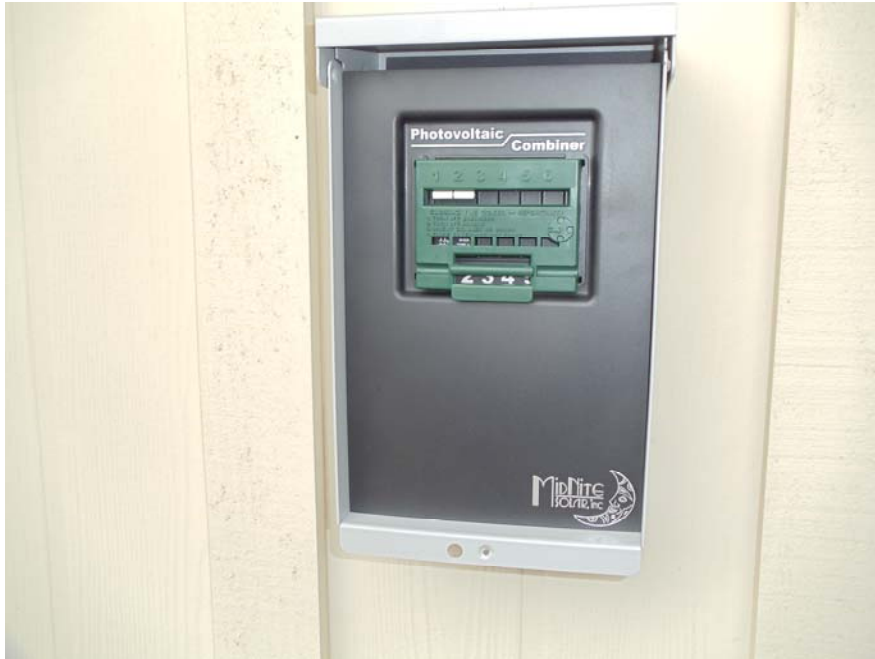
Figure 5 The black Deadfront with its integral green slider is snapped into place. Note breaker handles sticking through the slot at the top end on the slider. The green slider moves up and down based on exterior handle movement. This up and down action turns the breakers on and off. There is room for up to 6 breakers total. The MNPV6 Disco is ETL listed for 240VAC and 600VDC breakers in the same box. A 600VDC breaker will take up four more slots.
